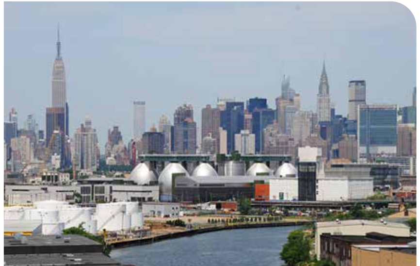
In the silver eggs, bacteria produce biogas from food waste and sludge for biomethane production.
