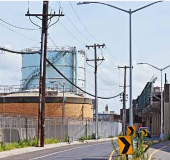
The wastewater treatment plant in Rockaway Beach currently flares biogas.
