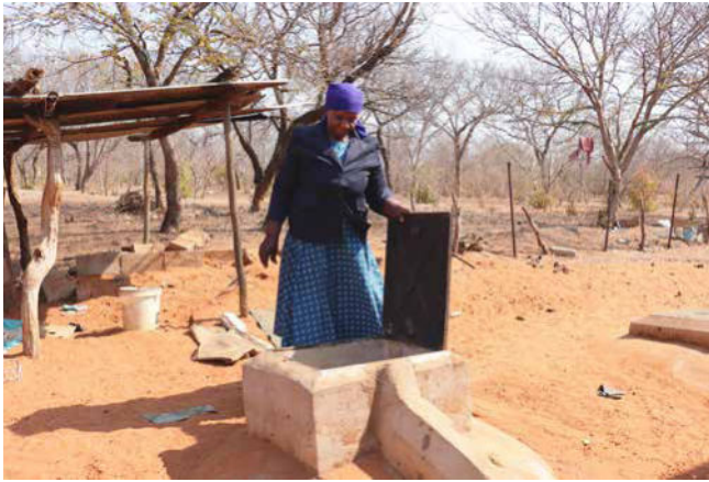
The manure mixed with water is being fed into the system here.
