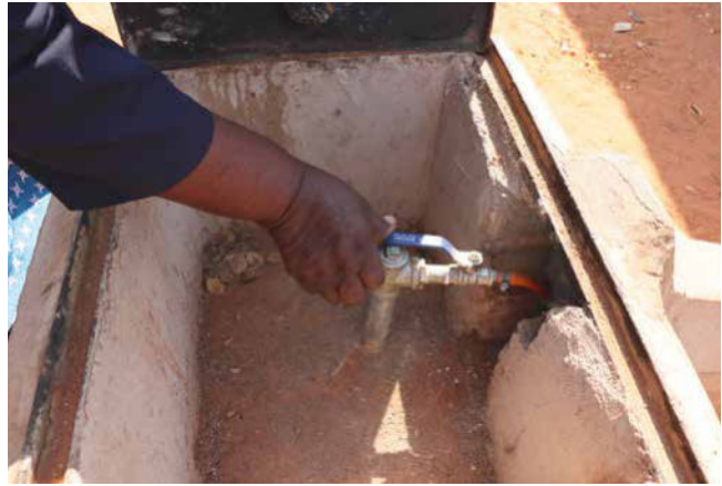
Above the digester is the gas tap, which the biogas farmer turns on when needed.
