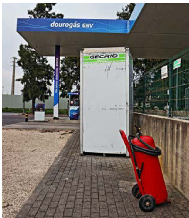
There are mobile biogas containers at this filling station. The bottled gas can be processed into biomethane on site and added to the other CNG.
